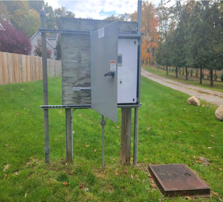
NOTES: Includes: wetwell, (2) 1.5hp pumps, scada, and controls.
