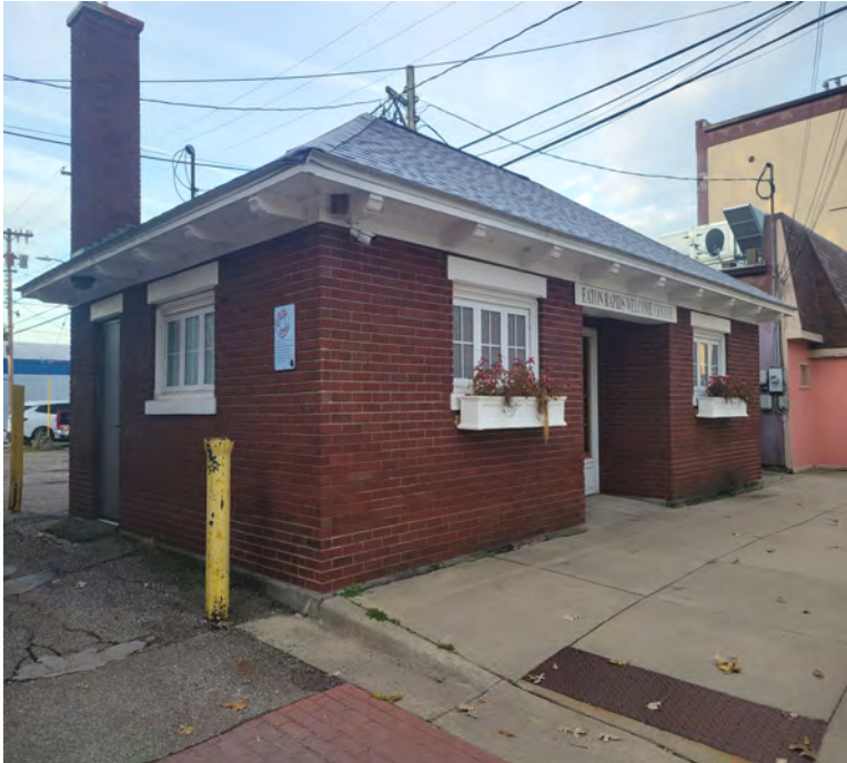
NOTES: Site improvements include: bollards.
