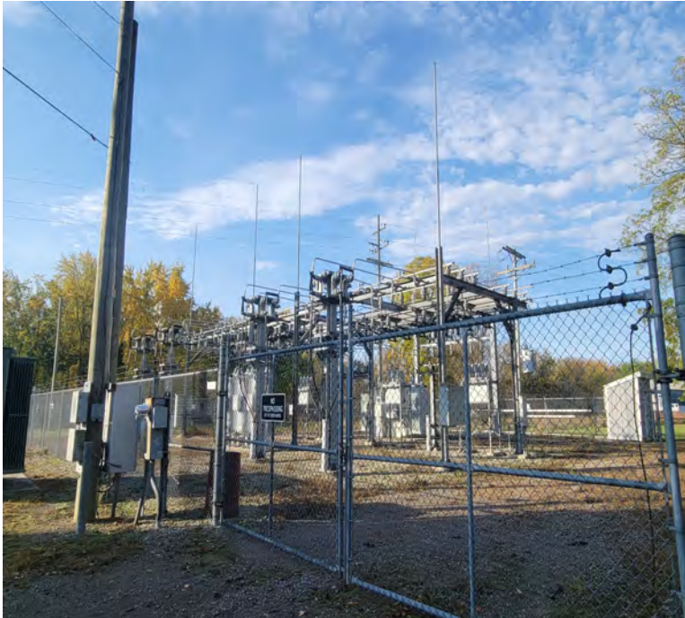
NOTES: 10,000 KVA rating. Includes: transformers, breakers, and grounding equipment. Site improvements includes: fencing.
