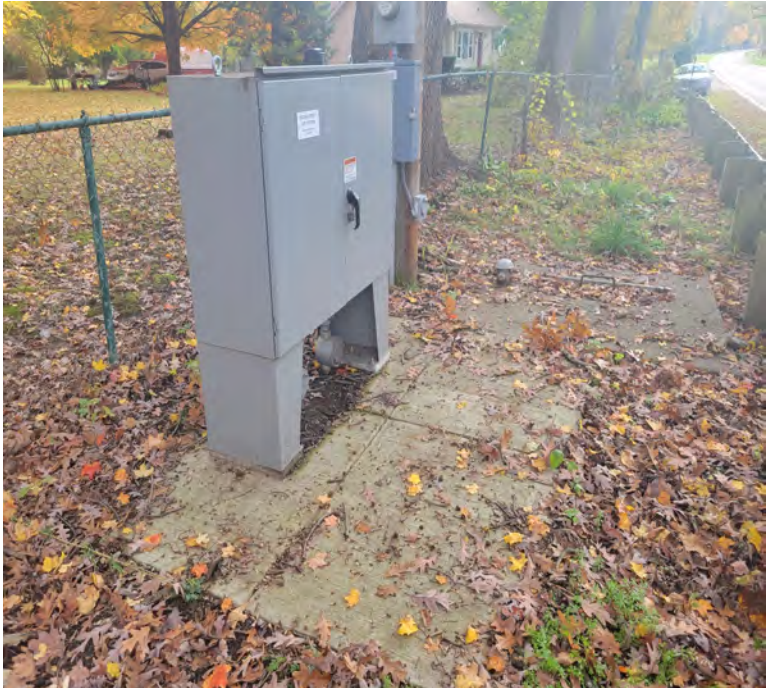
NOTES: Includes: controls, scada, wetwell, and (2) 1.5hp pumps.
